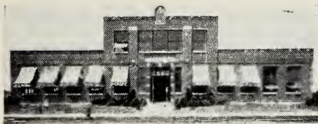
New Plant of the Haddon Press, Camden, N. J., Printers and Publishers (Printers of Harpers Magazine). This building was designed, built and equipped by The Austin Company
